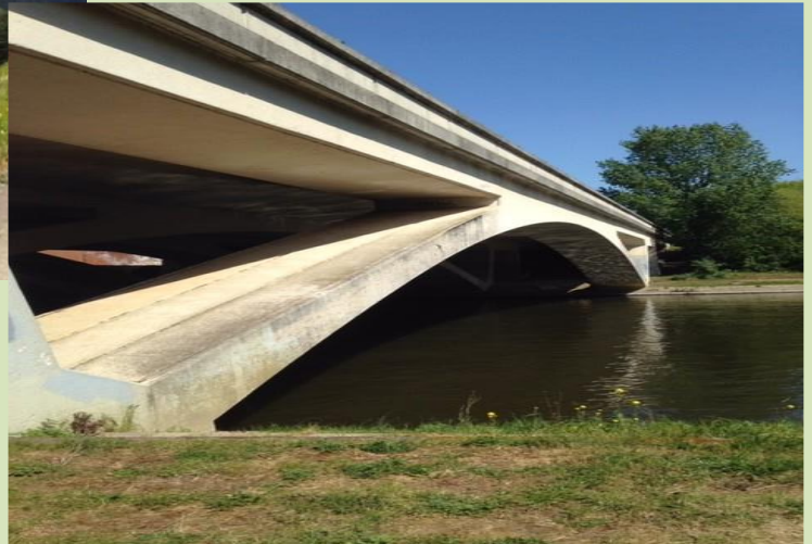
Sir Ove Arup's Single Span Road Bridge Over the Thames Photograph Dave Pope
